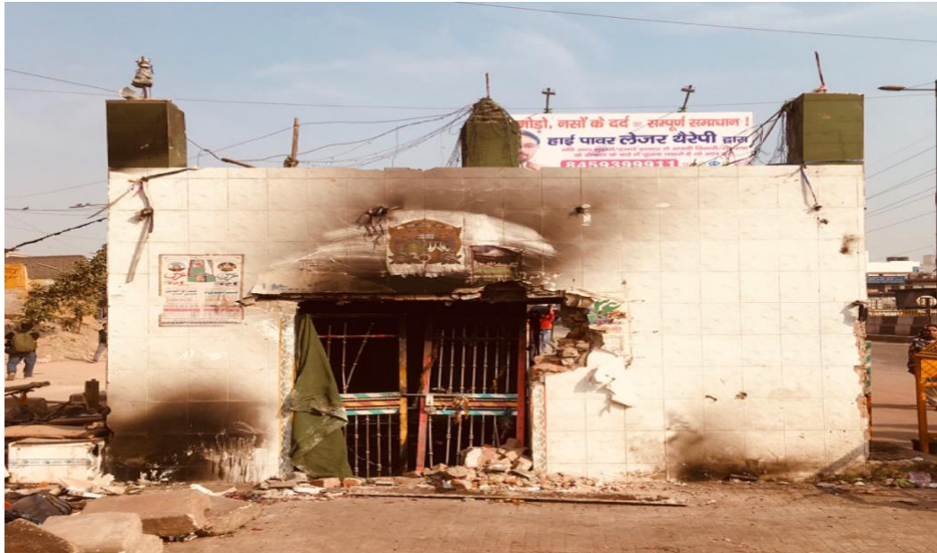
Burnt Mazar on Main Wazirabad Road: Feb 27, 2020
